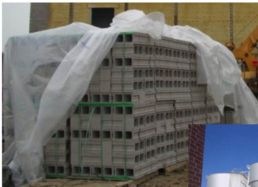
Store units and materials to produce mortar and grout off the ground and covered to keep them free from ice, snow, containments, and moisture intrusion.
