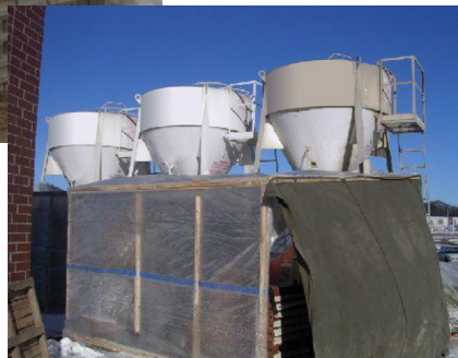
Store units and materials to produce mortar and grout off the ground and covered to keep them free from ice, snow, containments, and moisture intrusion.
