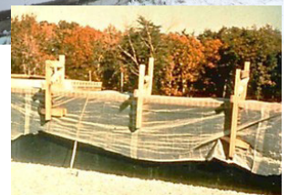
Insulating blankets may serve to meet both cover and heat requirements. When high winds are anticipated, hold downs may be needed to keep covers in place.
