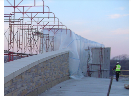
Enclosures are installed to suit project needs - multi-story as shown above or a small 'move-as-you-go' option shown at the right are just two options
