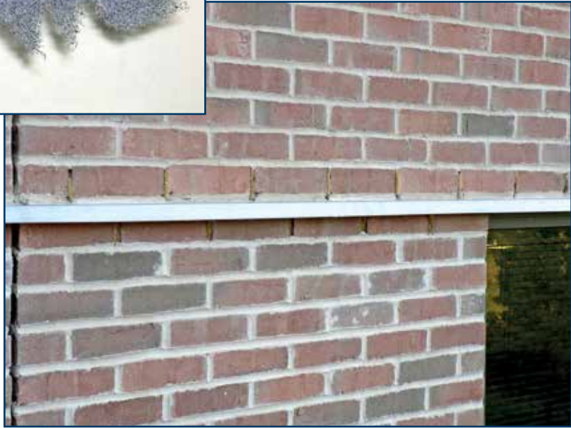
Figure 9 – Polymer mesh weep vents located 8 in. on-center for more drainage and drying capacity for this veneer replacement. The original unventilated veneer showed signs of distress after only eight years. Much of the water source in the wall cavity came from condensation of uncontrolled moist interior air from this densely occupied office building in a northern climate.
