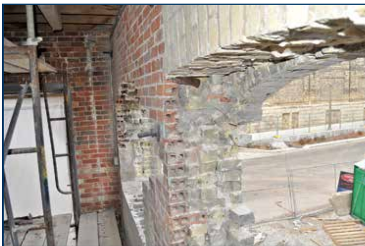
Figure 1 – Example of a mass masonry wall from the late 19th century.
