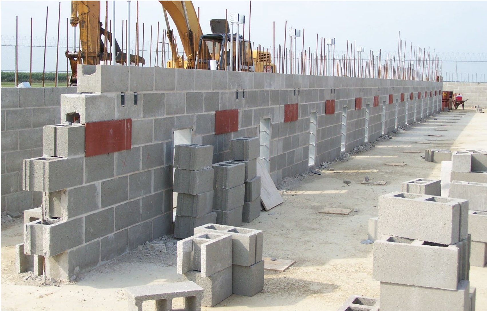
Heavily Reinforced Wall – Rushville Treatment & Detention Facility
