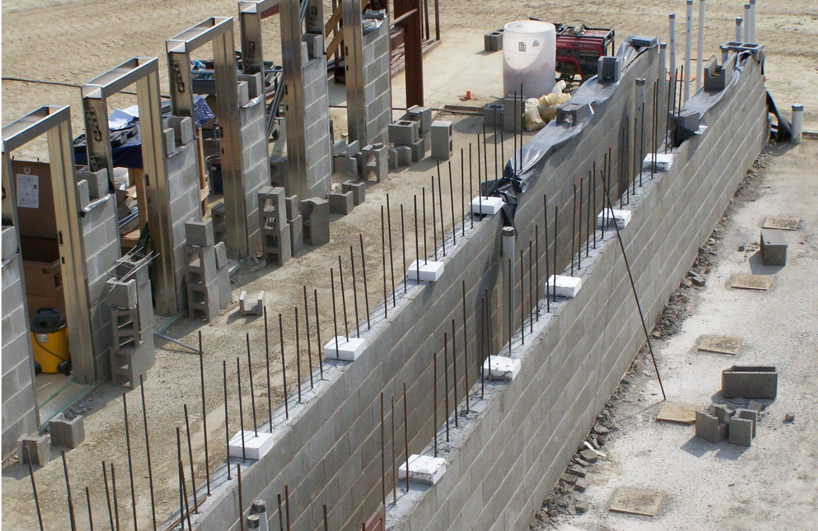
heavily reinforced wall – Rushville Treatment & Detention Facility
